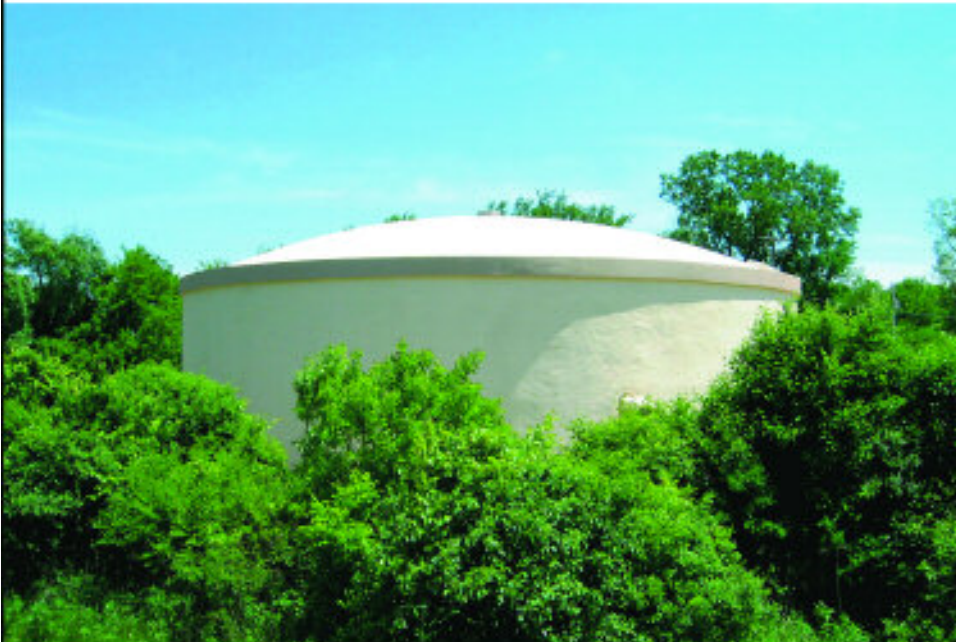
1.0 MG Natgun water tank for the Village of Poser, IL. Engineering by Robinson Engineering, Ltd., South Holland, IL.
